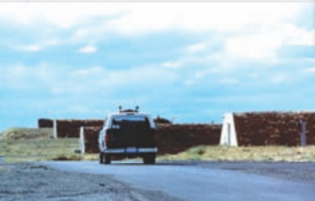
These “igloos” located in the U.S. Army’s Umatilla Chemical Depot house deadly chemical weapons like mustard gas. The igloos are usually covered with dirt to keep the inside cool for safety.
